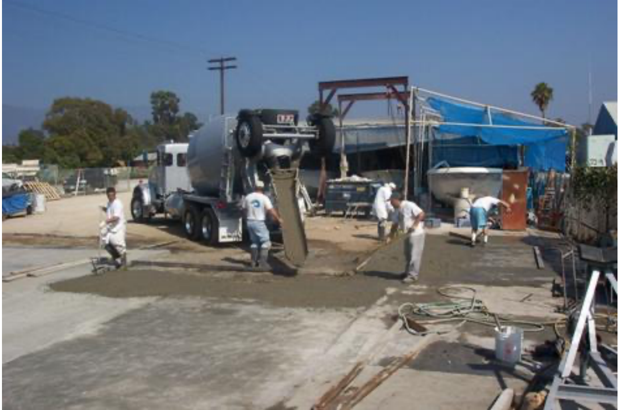
Above: The crew works diligently to pave the yard with concrete.
