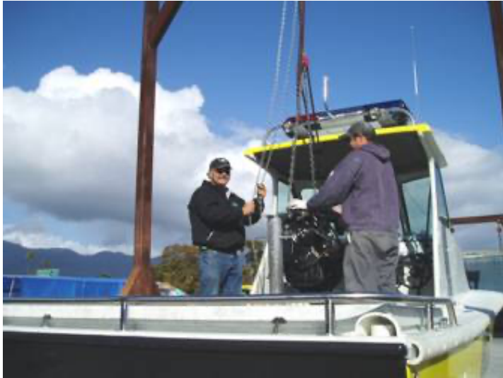
Don & Matt installing fire pump engine
